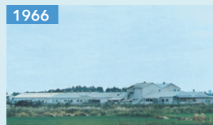
Construction of large-scale factory in Chiba
