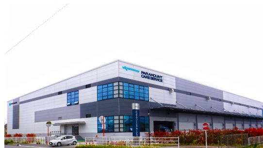
Atsugi Maintenance Center (opened in November)
